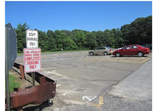
Parking spaces north of the school and near the baseball field can be replaced with porous asphalt to capture and infiltrate stormwater. A preliminary soil assessment suggests that the soils have suitable drainage characteristics for green infrastructure.
