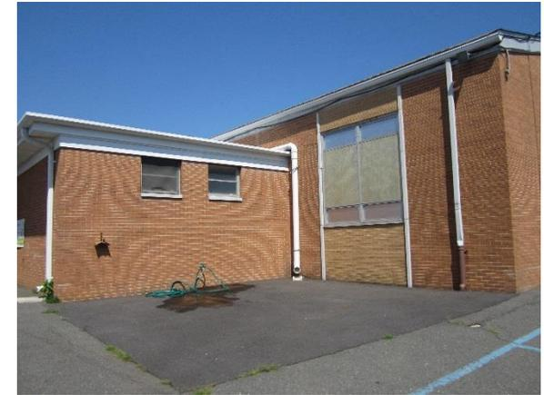
Parking spaces around the school can be replaced with porous asphalt to capture and infiltrate stormwater. A preliminary soil assessment suggests that the soils have suitable drainage characteristics for green infrastructure.
