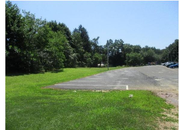
Parking spots and the existing asphalt playground can be replaced with porous asphalt to capture and infiltrate stormwater. A rain garden can be installed south of the parking lot to capture, treat, and infiltrate parking lot runoff. A preliminary soil assessment suggests that the soils have suitable drainage characteristics for green infrastructure.
